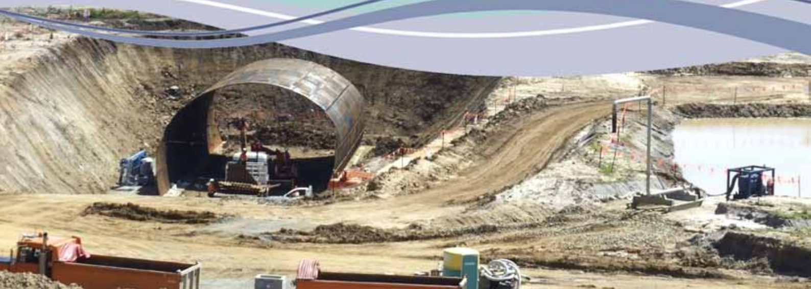
Construction tunnel under Cranbourne Road to assist with construction traffic.
