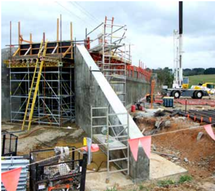
Derril Road underpass foundation.
