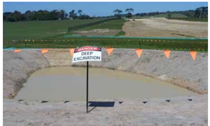
Sediment ponds have been constructed at locations along the alignment.
